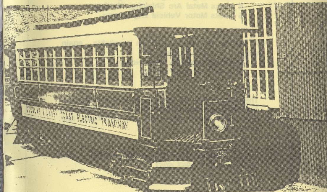
104 years old and still in service – Isle of Man Electric Tram No. 1 at Laxey.
